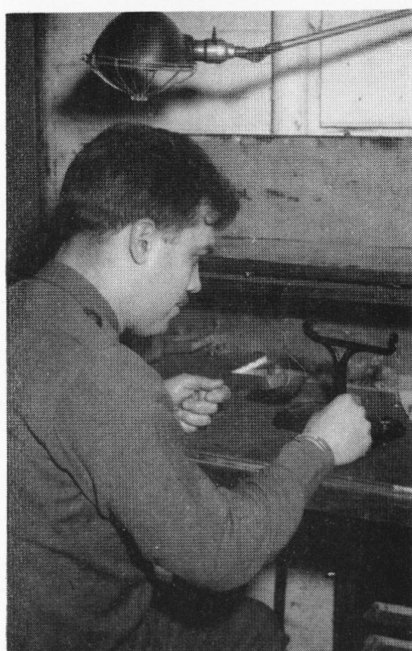
Using a grain scale, Joseph L. Macedo, an inspector in the Blanking Room, is spot-checking coin blanks for weight accuracy in accordance with U. S. Mint specifications.
